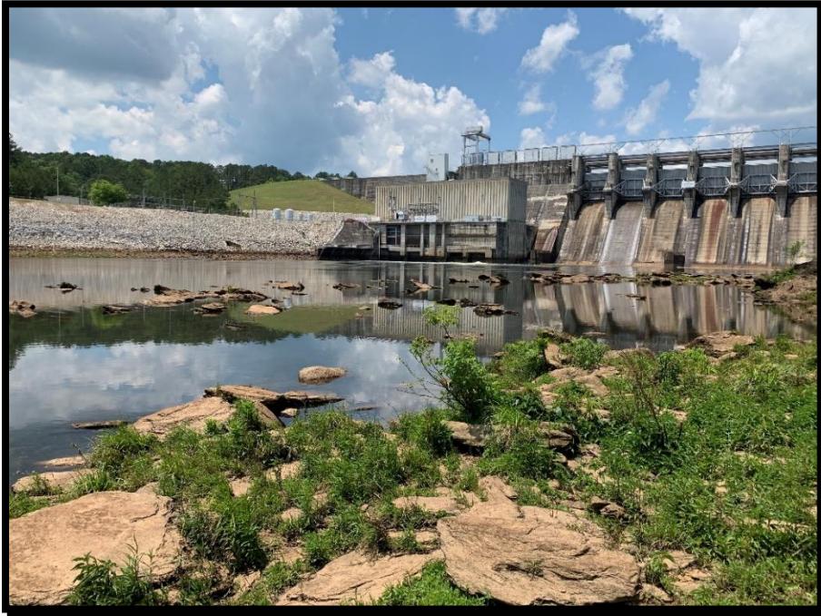
Figure 2: The Tallapoosa River below the R. L. Harris Dam.
