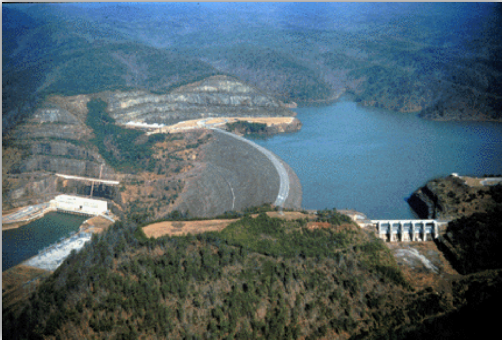
13 14 15 16 17 18 19 20 21 22 23 24 25 26 27 28 29 30 31 Figure 4-2. Carters Dam
