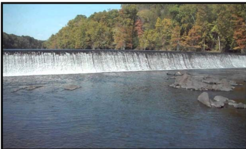
Example of Re-regulation Dam
