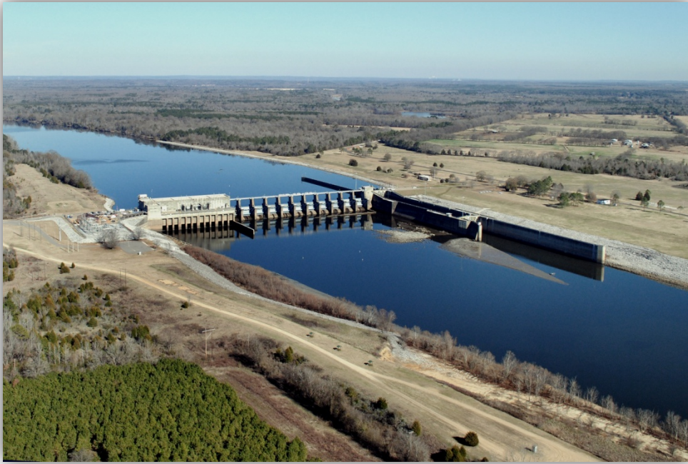
Figure 4-4. Robert F. Henry Lock and Dam
