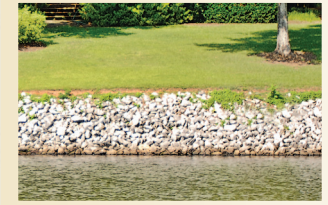
Riprap is the sloped piling of rocks 4-6 inches in diameter and is recommended for most shoreline stabilization projects.
